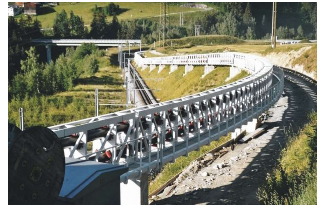
Cross-country Pipe Conveyors
