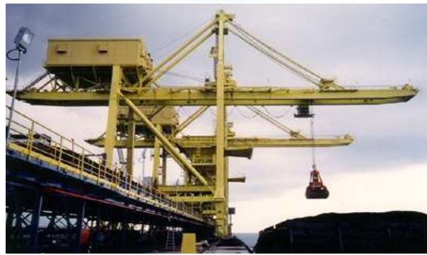
Ship Unloading System
